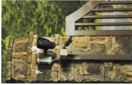
Electric & Existing Structure / Pole
