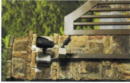
Electric & Existing Structure / Pole
