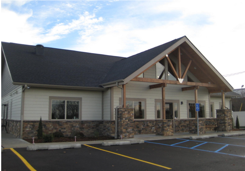
OWNER OCCUPANT MEDICAL OFFICE
